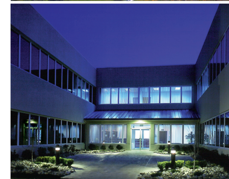
The original 1987 window installation on the left was matched in style and performance by the 1995 building addition on the right.
