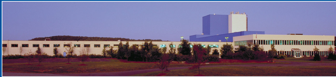
VEKA's own vinyl windows were installed in this Phase 1 construction and are still performing well after 25 years of service
