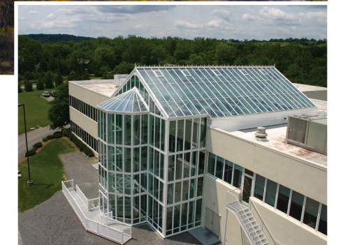
Constructed in 2005, this aluminum and steel reinforced PVC conservatory encloses a former parking area and is now a showroom space.
