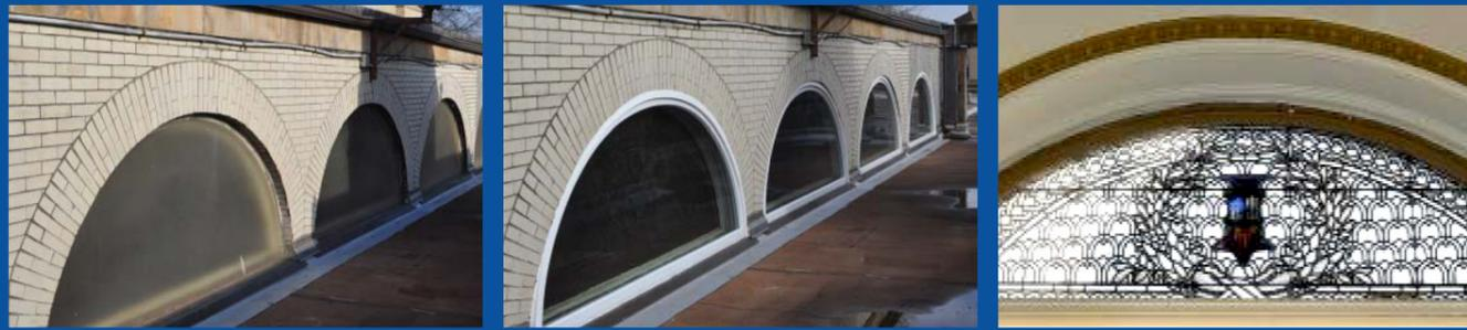
New vinyl fixed round tops protect stained glass windows from the elements while Argon filled IGs help prevent further color deterioration of the stained glass
