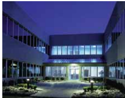
The original 1987 window installation on the left was matched in style and performance by the 1995 building addition on the right.
