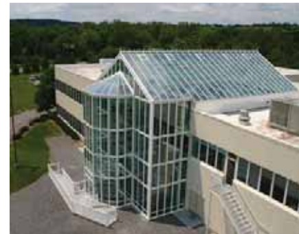
Constructed in 2005 this aluminum and steel reinforced PVC conservatory encloses a former parking area and is now showroom space.
